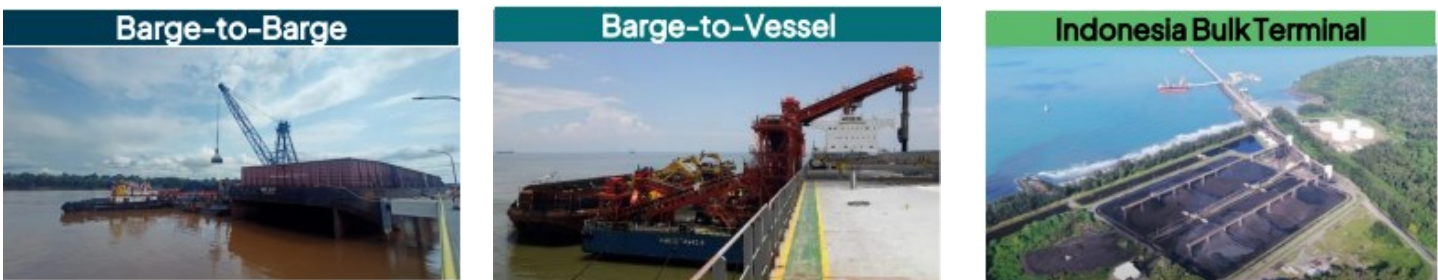
Figure 6. ADRO's Mineral Processing
