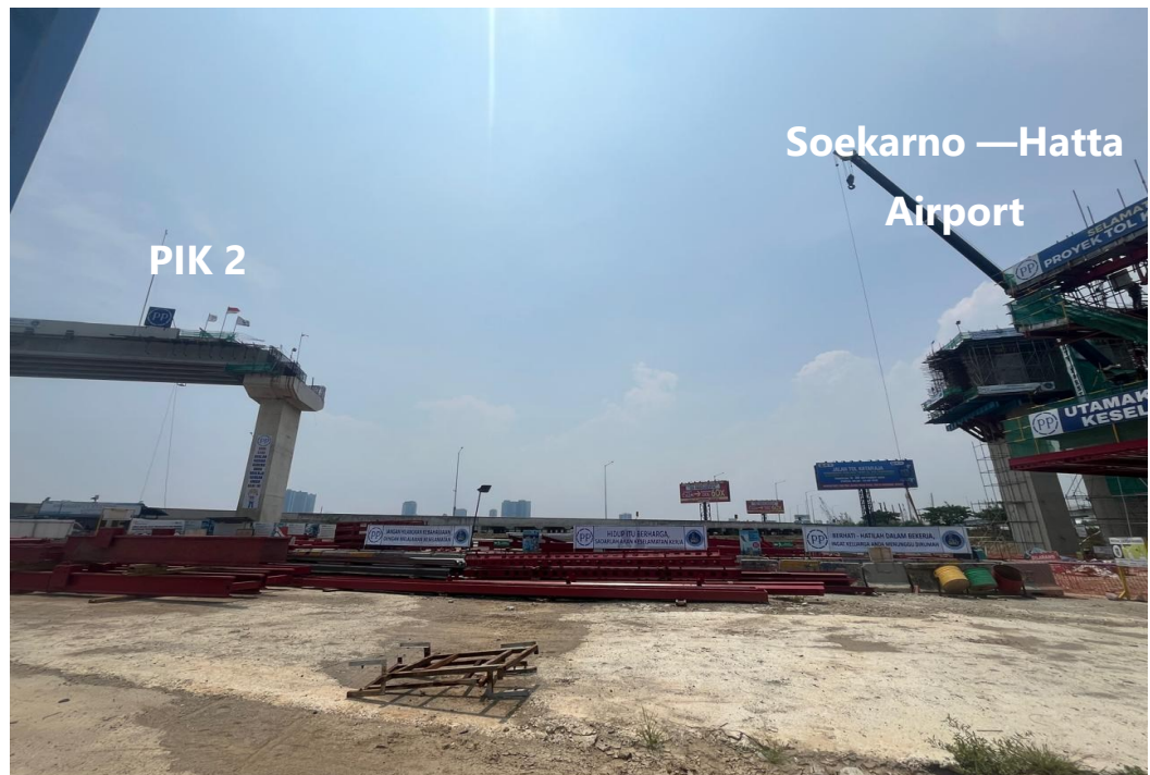
Figure 2. Junction Connection Progress – Linking PIK2 and Soekarno-Hatta Airport
