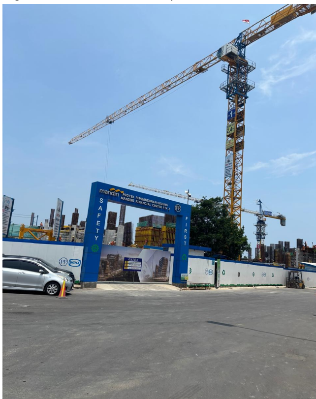
Figure 5. Mandiri Financial Center – Project Site Overview
