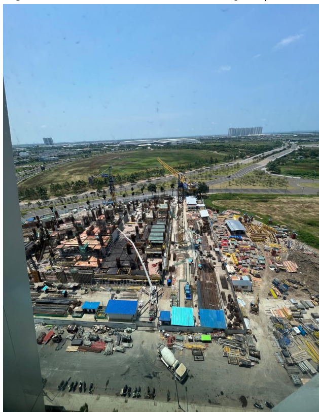
Figure 6. Mandiri Financial Center – Construction Progress Update
