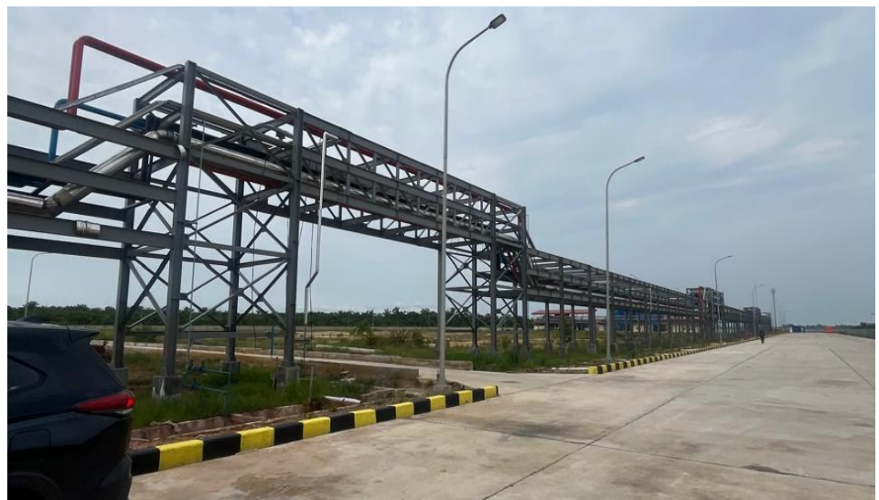
Figure 25. Pipeline Facilities from Plant and Storage Tanks to Jetty
